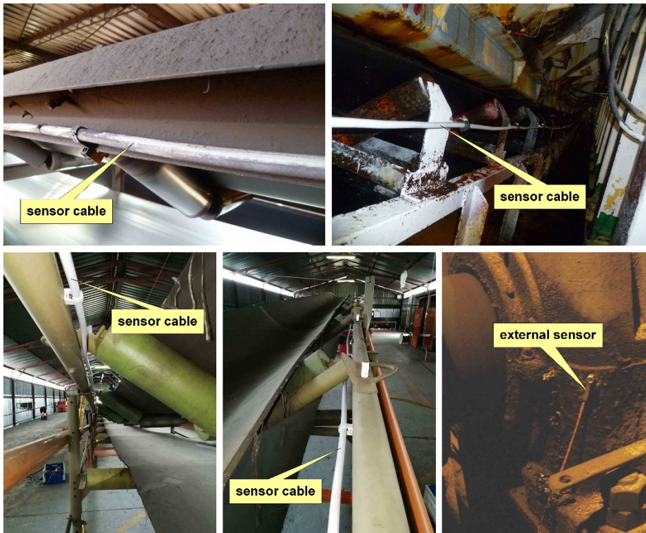
Figure 4 Temperature monitoring of idlers and other equipment
