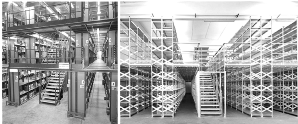
(a) Multi-tiered racking systems (b) Multilevel mezzanine warehouse
