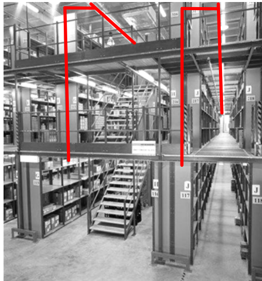
(a) Multi-tiered racking with mesh floor where one detector provides multilevel sampling
